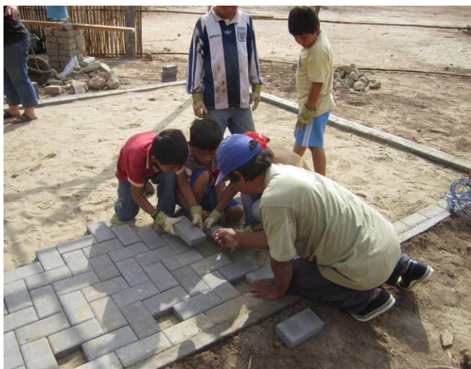
FIG 9: A few of the children learn how to lay out an interlocking stone platform
